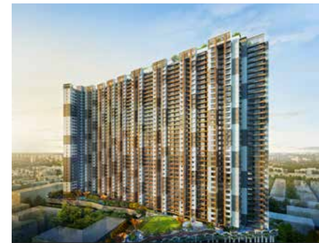
34 Park Estate, Goregaon (W)
